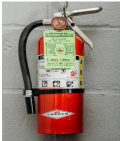
At least one tagged portable extinguisher of the 2A-10BC rating shall be mounted in the interior of the food truck/trailers.
