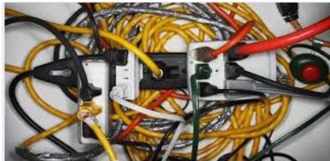
Extension cords shall not be utilized, nor are they a substitute for permanent wiring. Appliances shall be plugged directly into electrical outlets.
